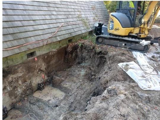
**Case Study 1:** Release of 240 gallons of fuel oil from outdoor tank. Cleanup of soil and groundwater resulted in more than \$300,000 in cleanup costs. The homeowner does not have insurance coverage for this release.
